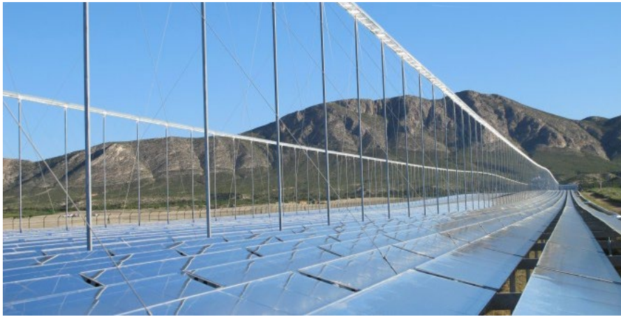
Figura 19. Sistema Linear Fresnel, Puerto Errado, Espanha. Fonte: World's Largest Linear Fresnel Solar Power Station Commences Operation | REVE News of the wind sector in Spain and in the world
